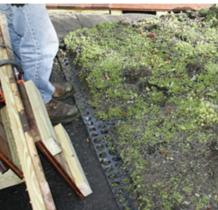
Figure 5. Vegetable planters and deck sections built with ipe were installed on top of the slip sheet (top). Next, the one-meter-square roof panels were cut to size with a cut-off saw and fitted in place (above). The “eggcrate” water reservoir on two sides of each panel was left exposed (left) so that the panels could interlock.
