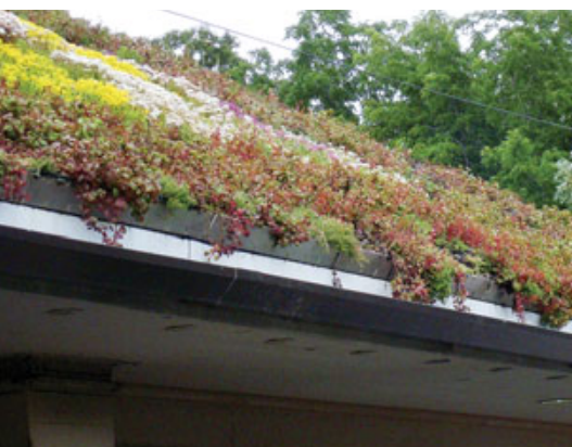
Figure 2. GLT roof panels are available for virtually any roof pitch. On this green roof, L-shaped aluminum brackets taped to the waterproofing layer finish the panel edges and help prevent wind uplift.
