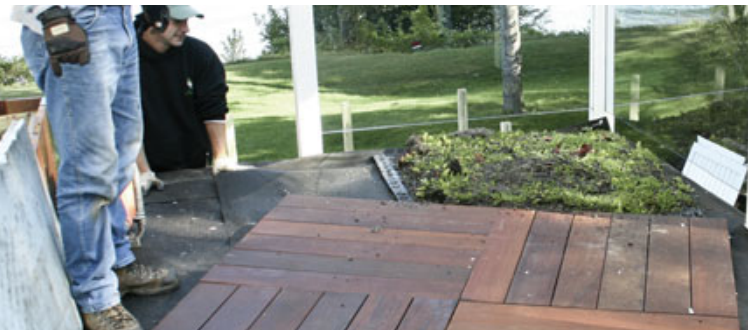
Figure 5. Vegetable planters and deck sections built with ipe were installed on top of the slip sheet (top). Next, the one-meter-square roof panels were cut to size with a cut-off saw and fitted in place (above). The “eggcrate” water reservoir on two sides of each panel was left exposed (left) so that the panels could interlock.
