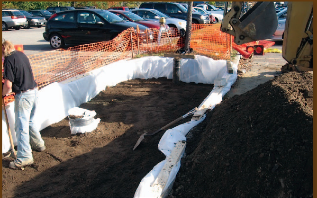
FIGURE 3-4 Bioretention retrofit installation at the University of New Hampshire, 2008
