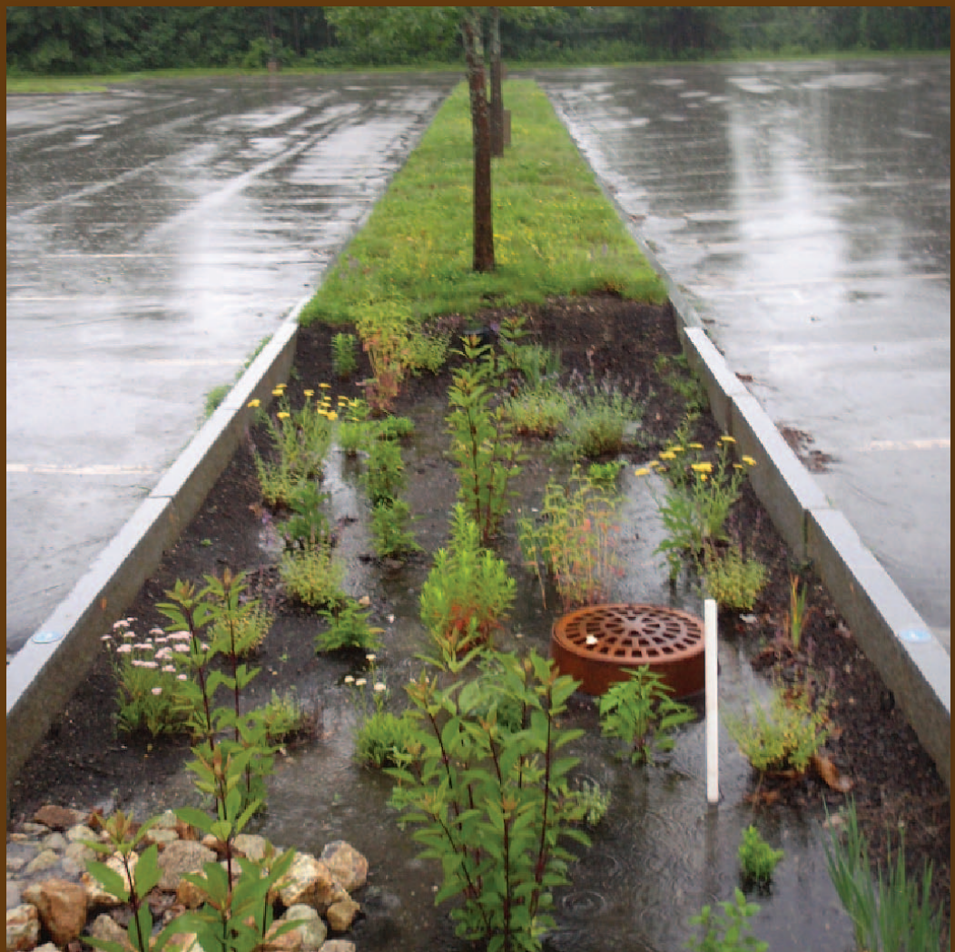
FIGURE 3-5 Completed Bioretention Retrofit Installation 2008
