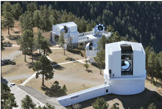
Apache Point Observatory. Pictured left to right are the 0.5 meter telescope, the 2.5 meter Sloan Foundation Telescope, the New Mexico State University 1 meter telescope, and Astrophysical Research Consortium 3.5 meter reflector.
