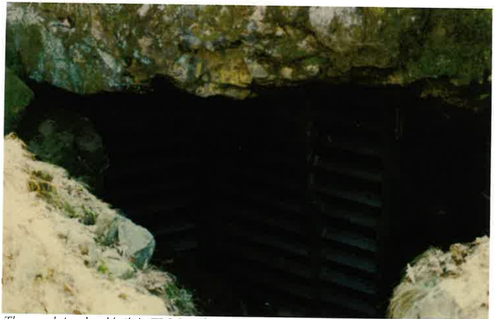
The gates designed and built by TROG are bat friendly. Both the rare and common bat species that use this cave can fly between the bars of the gate.
