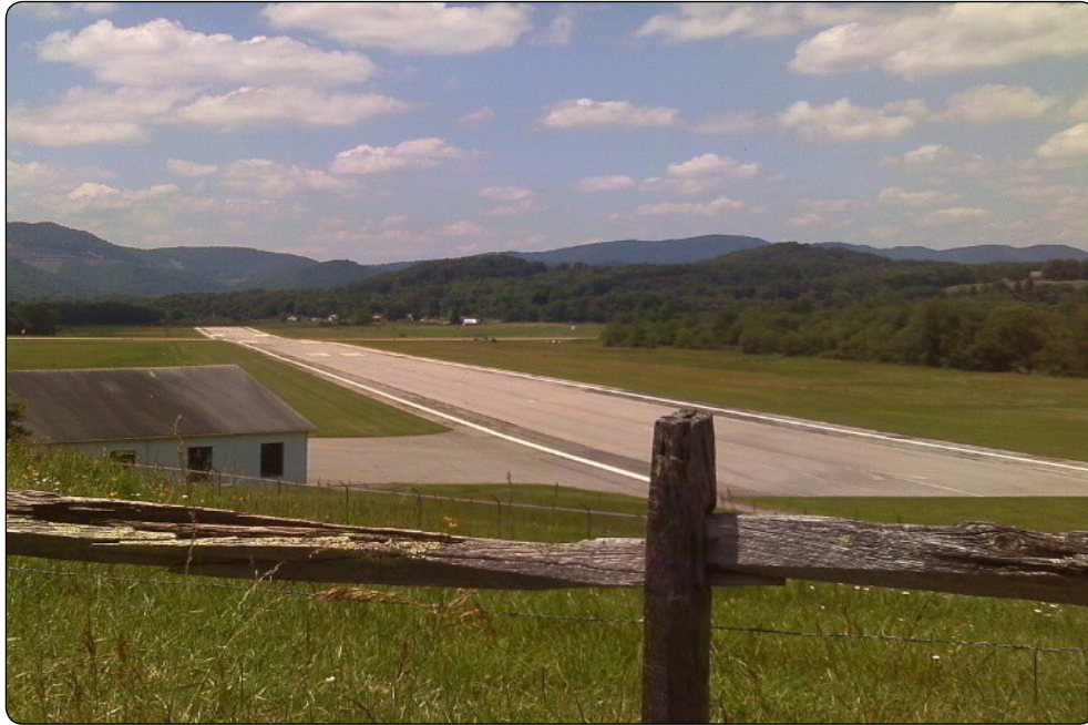
Figure 3-4. Elkins, WV airport.
