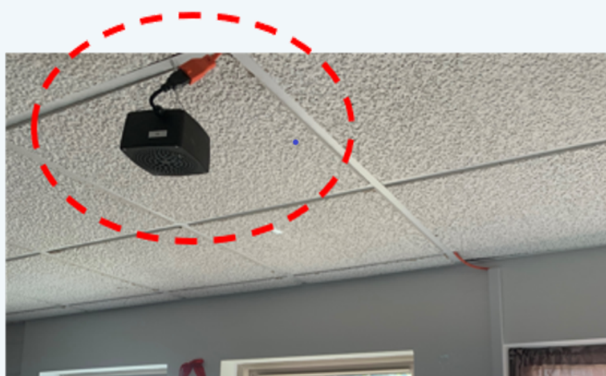
(A) Continuous air quality monitoring via wireless sensor
