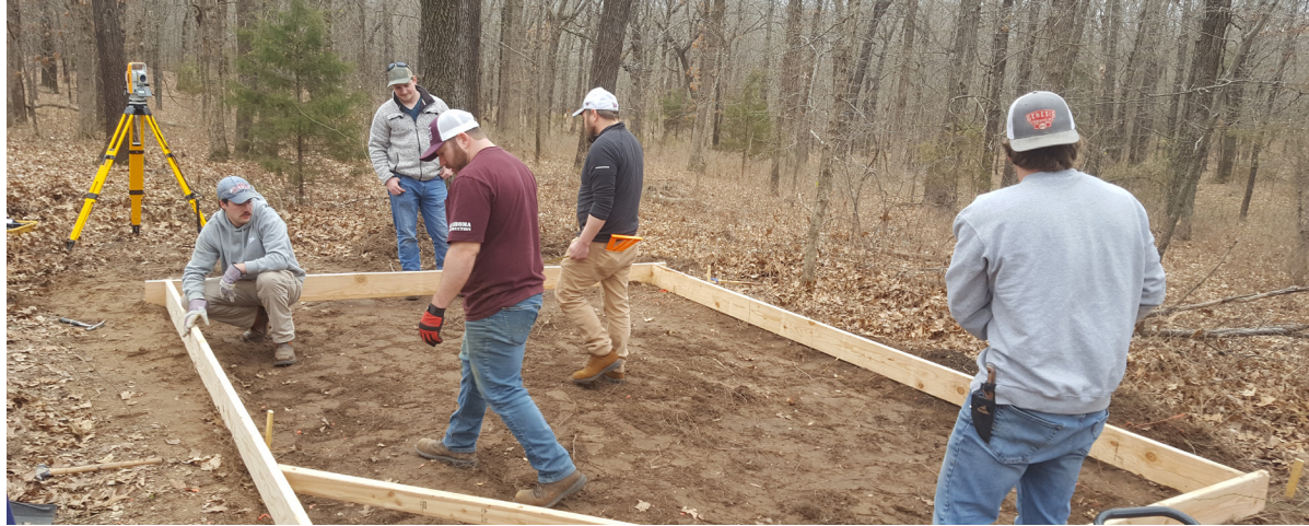
Laying Out the Foundation
