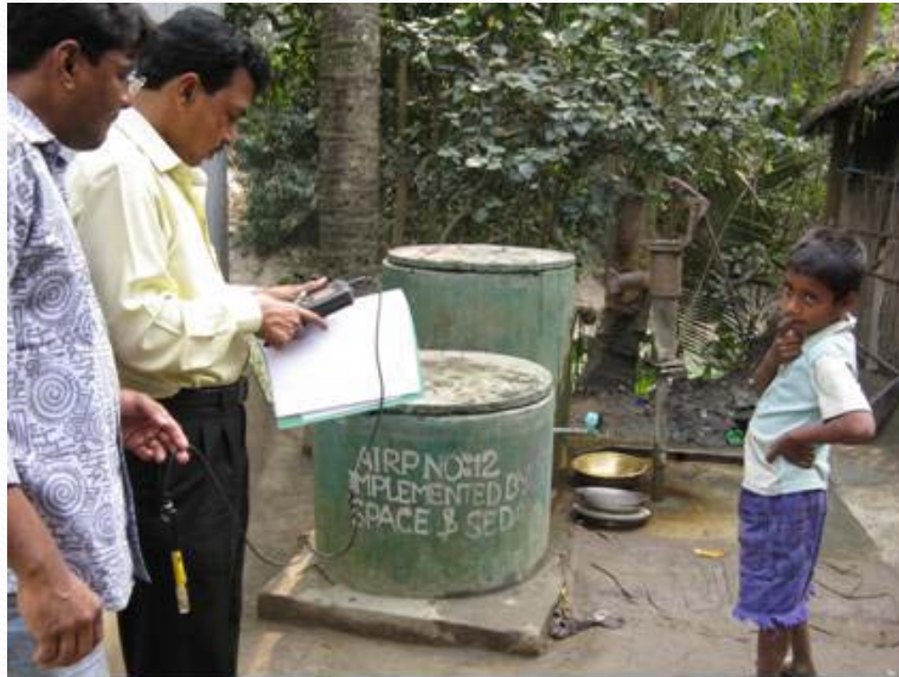
2-Chamber SEDA Plant
