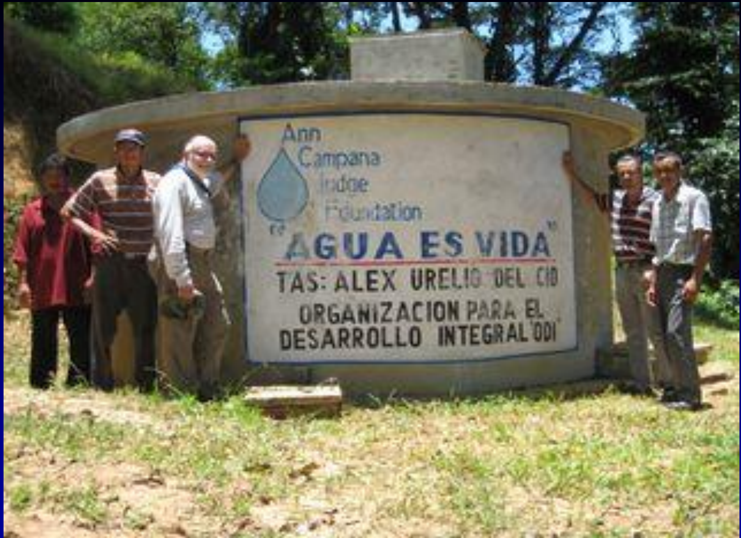
Tank at Brisas del Rio Cuyamel
