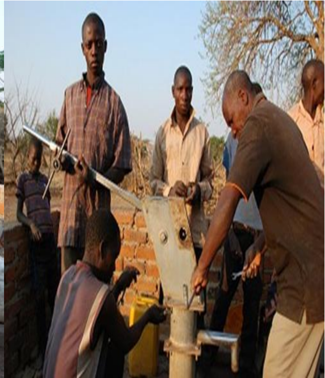
A Pump Minder repairing and training youth on pump repair and
